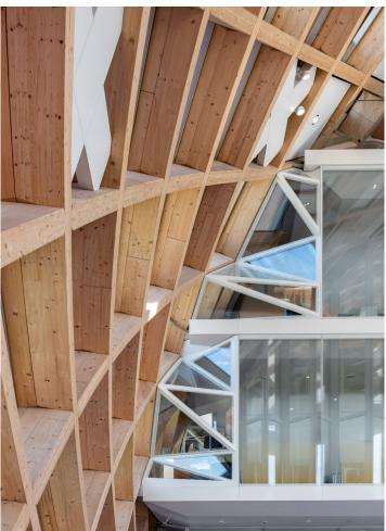
Using a sophisticated plug-in principle, the individual beams were fitted to each other perfectly. Since the timber grid shell of the Swatch building serves as a large office façade, it also had to meet various technical requirements. A complex network of cables is discreetly integrated into its structure.
